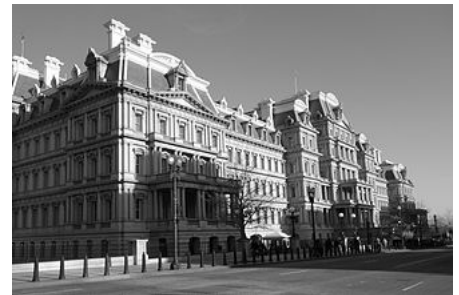
Eisenhower Executive Office Building, built in 1888 in Washington, DC
