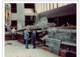
July 17: Hyatt Regency walkway collapse
