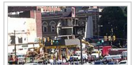
June 5: Rescue operations on the afternoon of the collapse.
